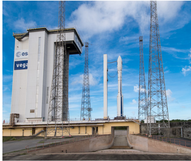
Figure 1.4: Launch platform of Vega in Kourou, French Guiana. View on the exhaust duct to be covered by a sonic crystal.
